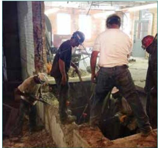
Workers jackhammer through the lower level of the administration building as part of the construction of an elevator shaft. The new elevator will service all four floors of the building.
